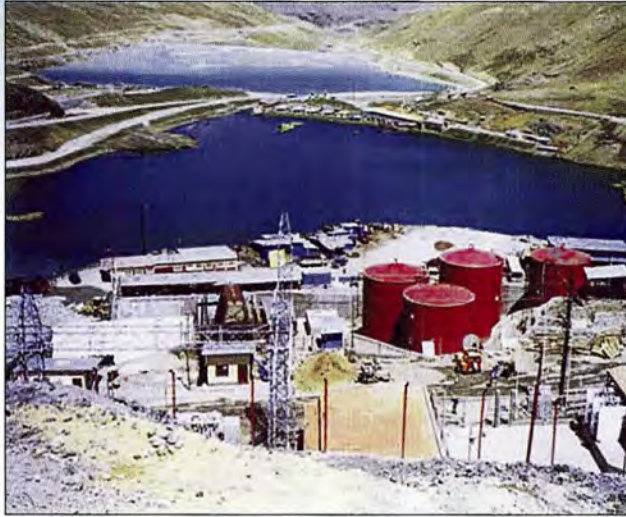
Central Térmica de San Rafael (Minsur). San Rafael Thermal Power Station (Minsur)
