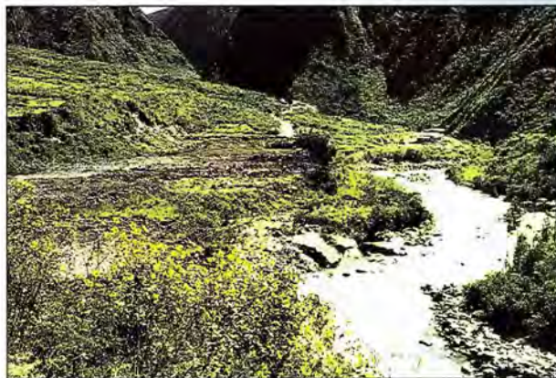
Chuan - Zona donde se construyeron las Obras de Cabecera. Chuan - Area where the Head Works were built.
