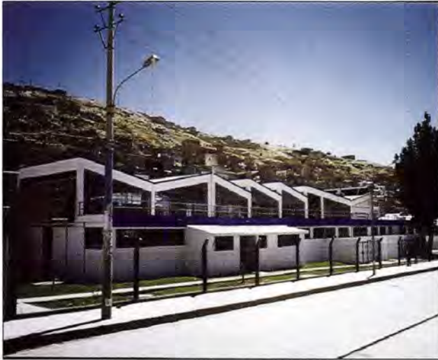
Vista exterior de la C.T. de Bellavista. External view at the Bellavista Thermal Power Station
