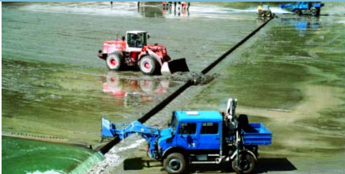
Limpieza del Embalse - CHSGBII / Reservoir cleaning. SGBII PS.
