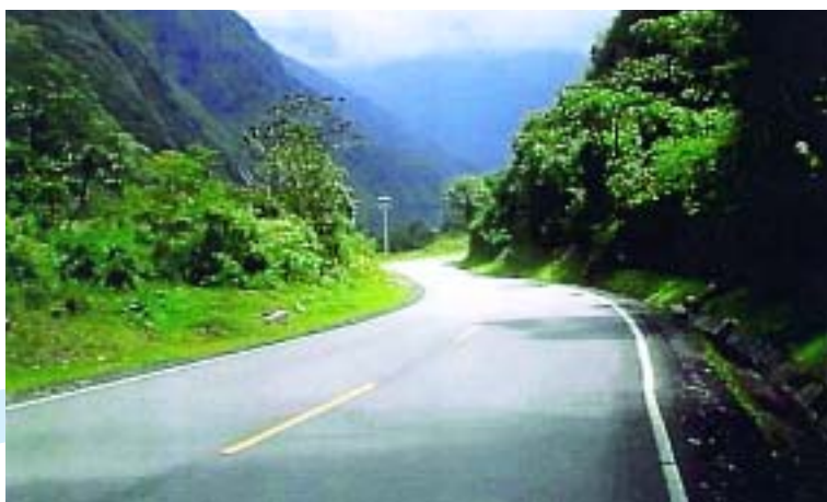
Carretera Tabinapampa - Tunquini: Sector Chuani Tabinapampa - Tunquini Highway: Chuani Sector
