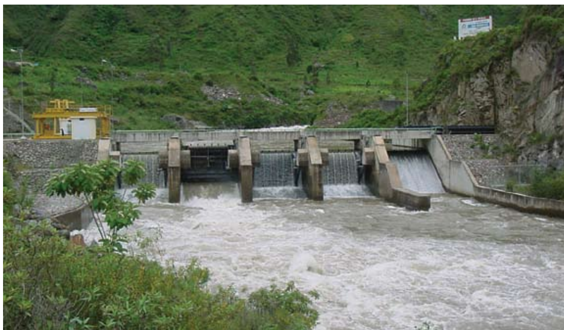
Presa derivadora del sistema de captación C.H. San Gabán II Diverting reservoir of the water collecting system, San Gabán II Hydroelectric Power Plant
