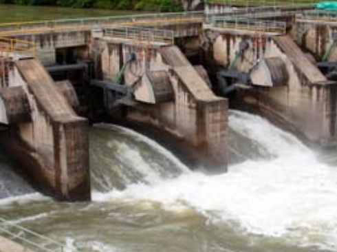
Presa derivadora del sistema de captación C.H. San Gabán II Diverting reservoir of the water collection system at San Gabán II Hydroelectric Power Plant
