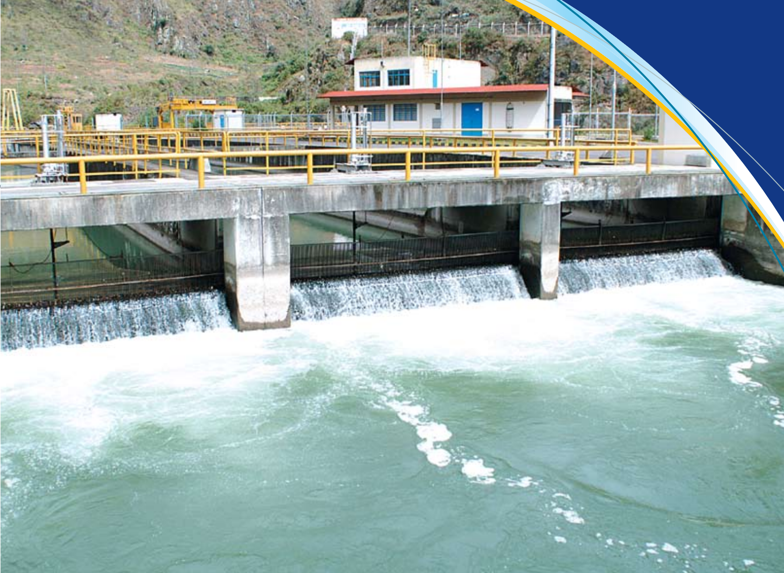
Naves desarenadoras C.H. San Gabán I Water settlement pond, San Gabán II Hydroelectric Power Plant
