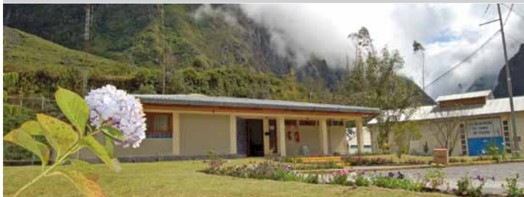
Oficinas administrativas C.H. San Gabán II / Administrative offices at San Gabán II Hydroelectric Power Plant
