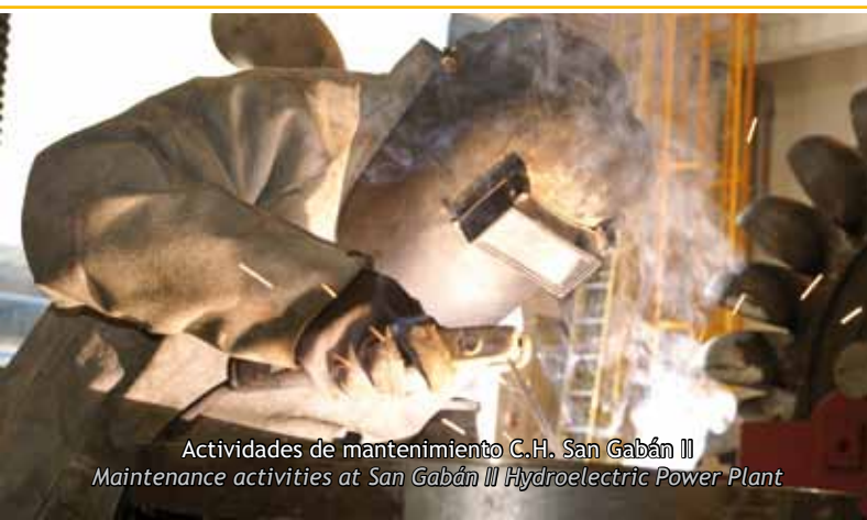
Mantenimiento válvula esférica No 1 C.H. San Gabán II Nr. 1 spherical valve maintenance at San Gabán II Hydroelectric Power Plant
