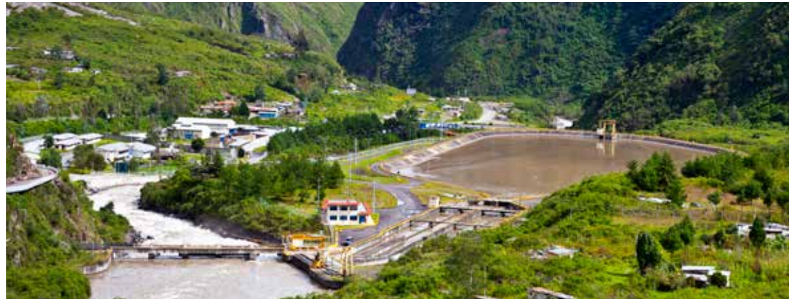
Río San Gabán, bocatoma y embalse regulador. Chuani. San Gabán river, water inlet and regulating dam. Chuani.
