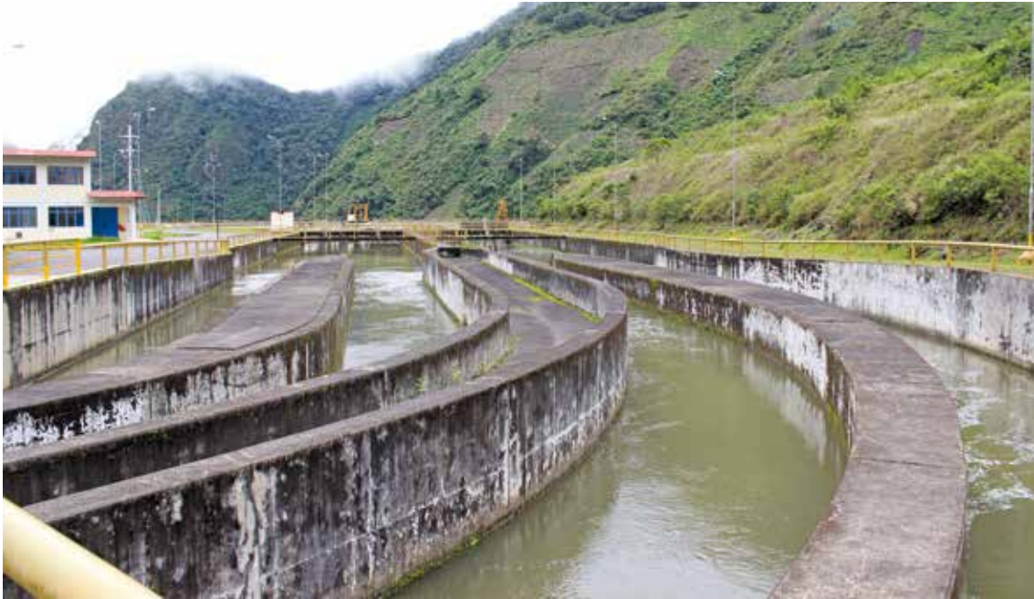
Sistema de Desarenadores C.H. San Gabán II / San Gaban II Hydroelectric Station desander system
