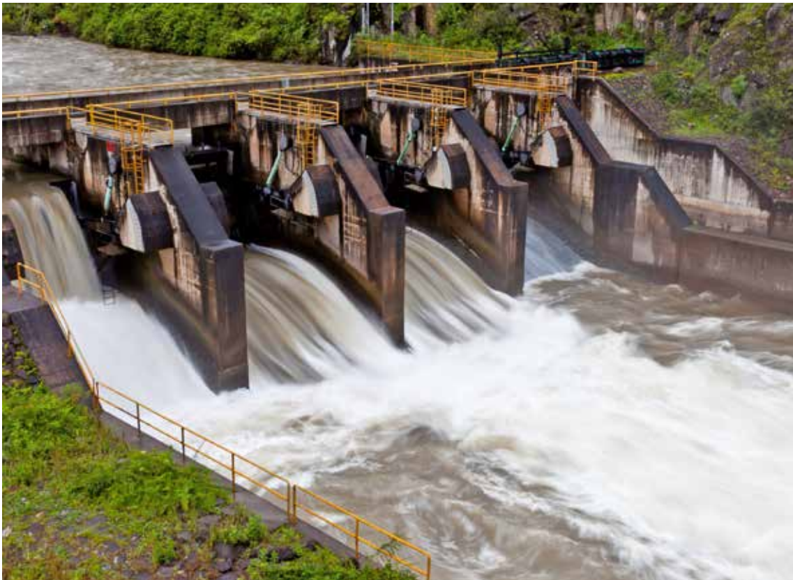
Bocatoma C.H. San Gabán III / San Gaban III Hydroelectric Station intake
