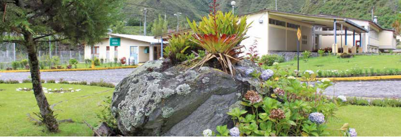
Instalaciones Villa de Residentes C.H. San Gabán II / San Gabán II Hydroelectric Station Village facilities
