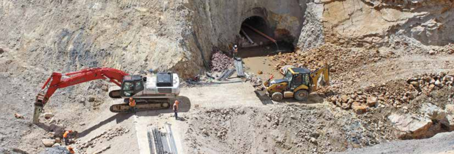
Obras Presa Pumamayo (32 MMC) / Works at Pumamayo dam [32 MMC]
