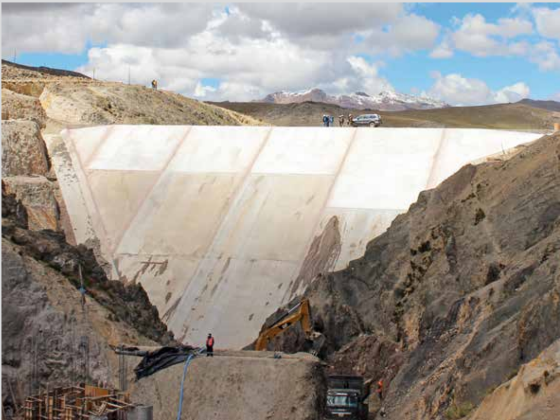
Presa Pumamayo (32 MMC) Talud aguas arriba / Pumamayo dam [32 MMC] upstream slope
